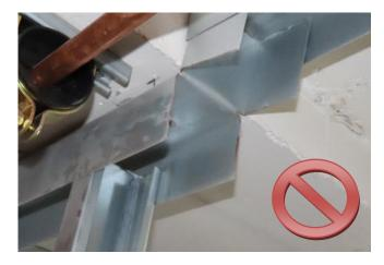
The flange(s) must be restored via framing angle or strapping— same gauge.
